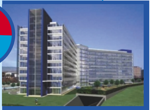
2 ■ SILab was commissioned by Sulzer Infra Romandie to assess the effect of various types of solar protection on an office building at the Geneva-Cointrin airport. The example shows the energy distribution in summer with black solar protection.
